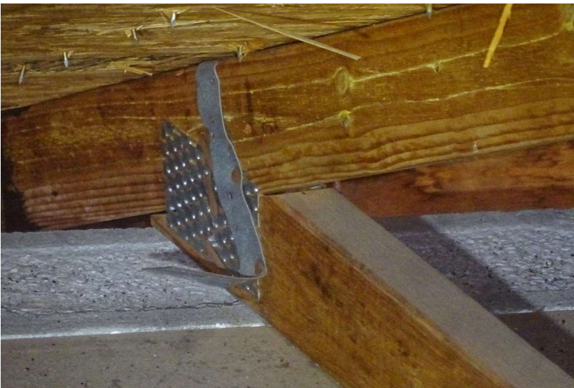
Single wrap with at least 2 nails in the embedded side and at least 1 nail in the wrapped side
